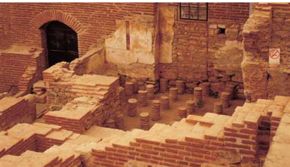
Below: Baths with stilted floor. At Ephesus, the Baths of Varius were located just off Curetes Street. The limited excavations have revealed a changing room, a frigidarium (for a cool bath), a tepidarium (for warm baths), a caldarium with its heated floors (shown), and a sudatorium (sweat room).
